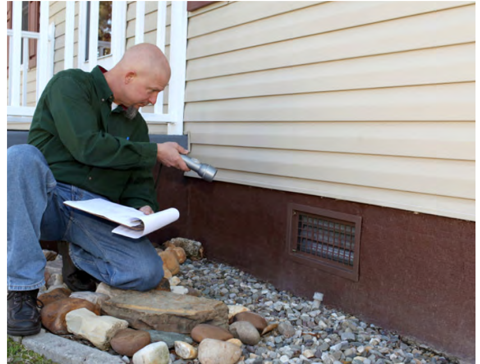
Figure 15. Home inspector checking maintenance systems.
