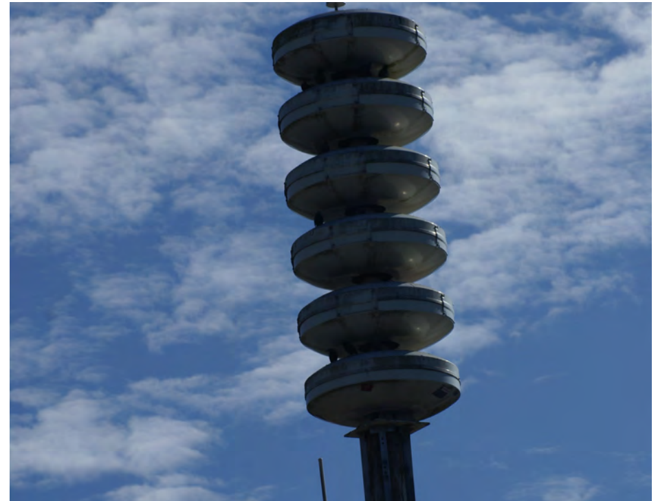
Figure 41. All Hazard Alert Broadcast siren and light tower.
