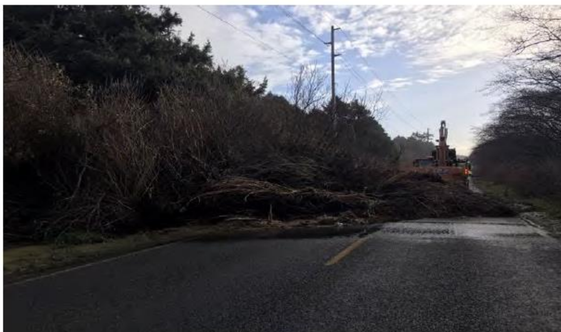
Figure 4-2 December 18, 2018 Mudslide at MP 33.5
