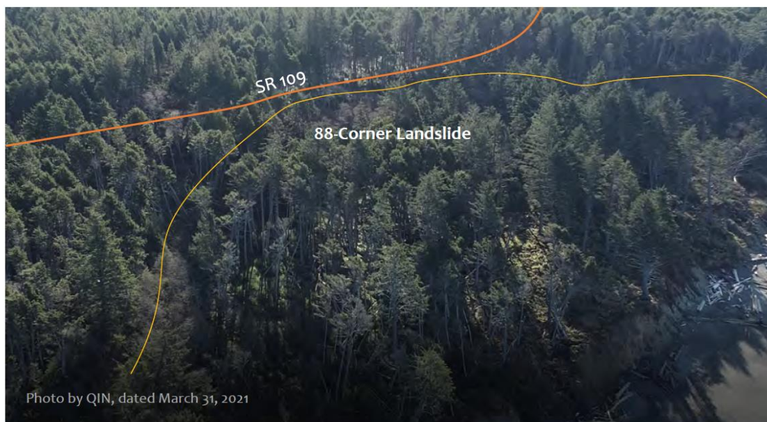
Figure 9-12 Proximity of 88-Corner Landslide to SR 109
