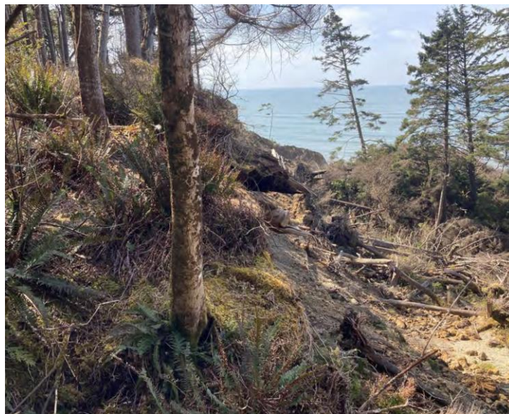
Figure 9-13 88-Corner Landslide Along SR 109
