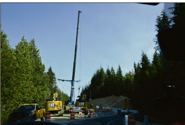
Approaching culvert work area.
