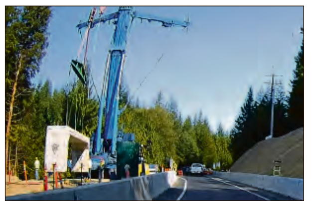
A culvert section about to be lowered into place.
