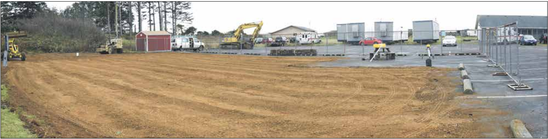
The site of the former court house, which was destroyed in a fire on October 15th, has been cleared as of December 6th. Four modular units (in the background) will be placed here as a temporary facility until the permanent court house can be built in the relocation area just across the street from the Roger Saux Health Center. Photo by Larry Workman
