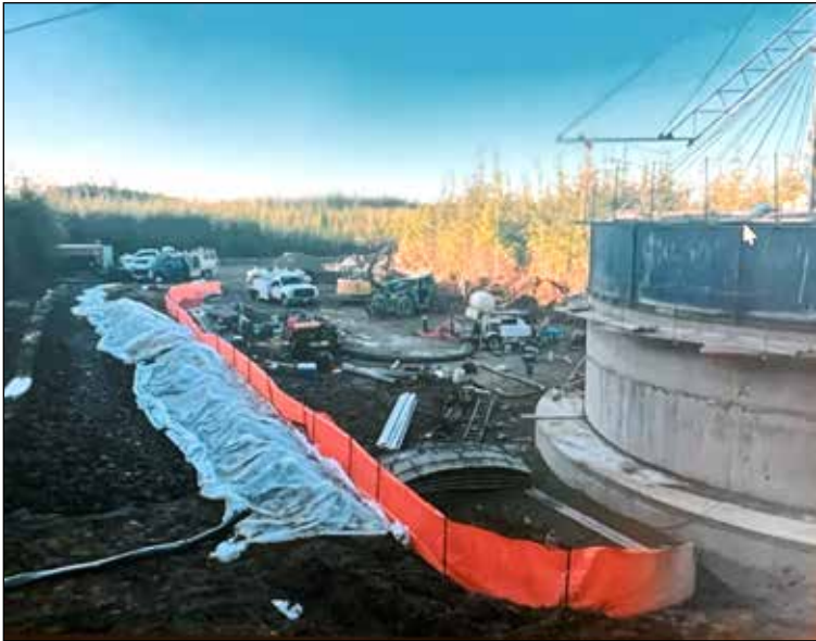
Photo of the Taholah water tower being constructed. Photo by Wenaha Project Management team.
