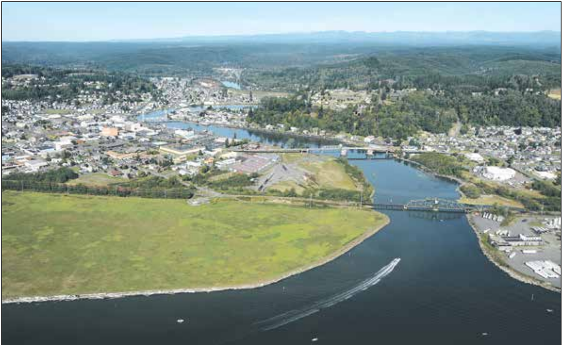
Levees along the Hoquiam River were to provide protection from high water. Photo by Larry Workman
