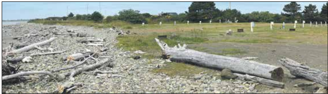
There is extensive erosion at the Quinault RV Park. Photos by Larry Workman
