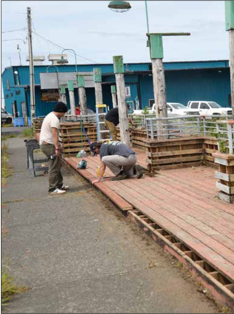
The boardwalk between the fishhouse and the Riverside Fitness Center under repair on June 19 by Hultman Construction & Environmental Inc. Photo by Larry Workman
