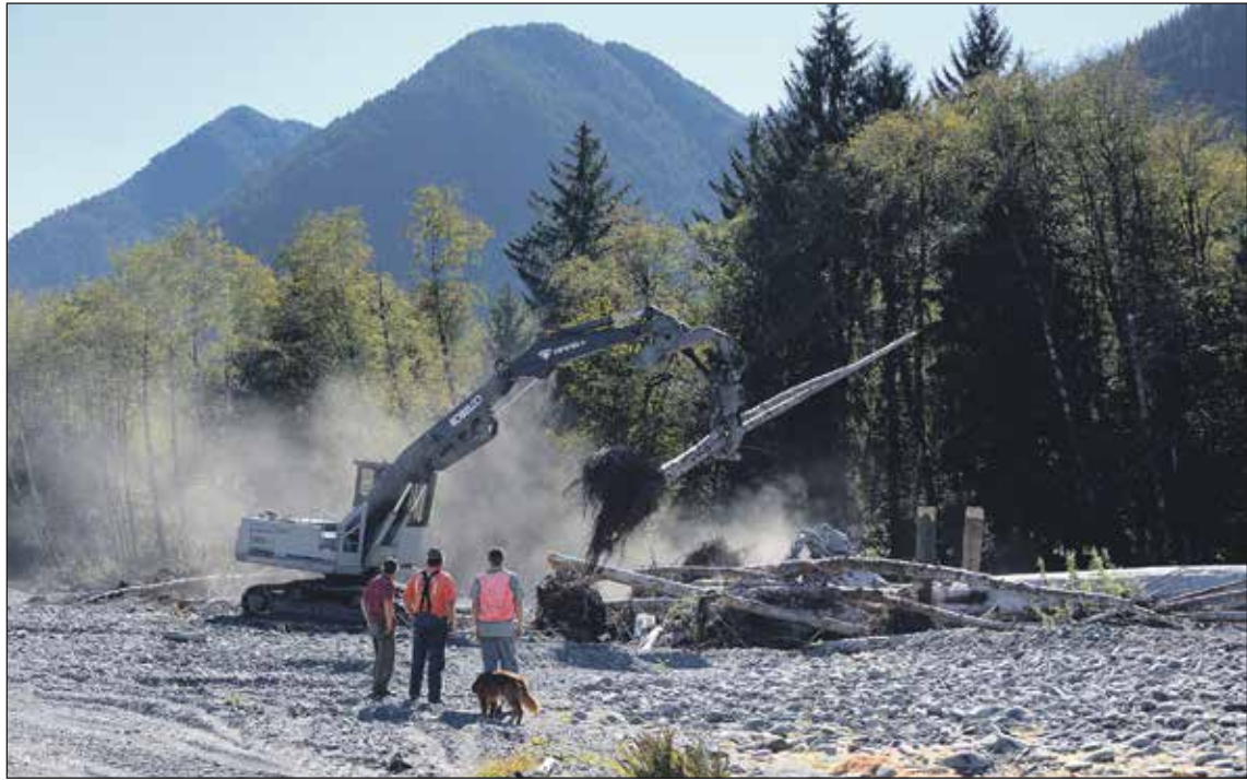
Engineered log jam work near the Wilson's Slough reach on the Quinault River in September 2019. Photo by Larry Workman
