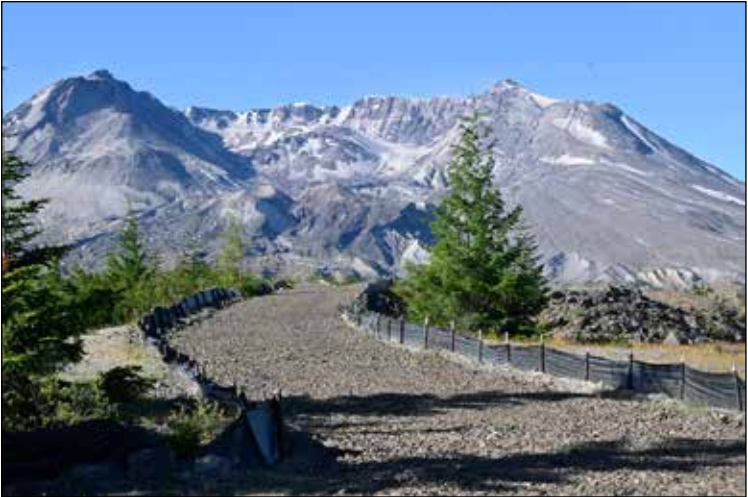
A section of the road being built to access Spirit Lake and the Intake tunnel.
