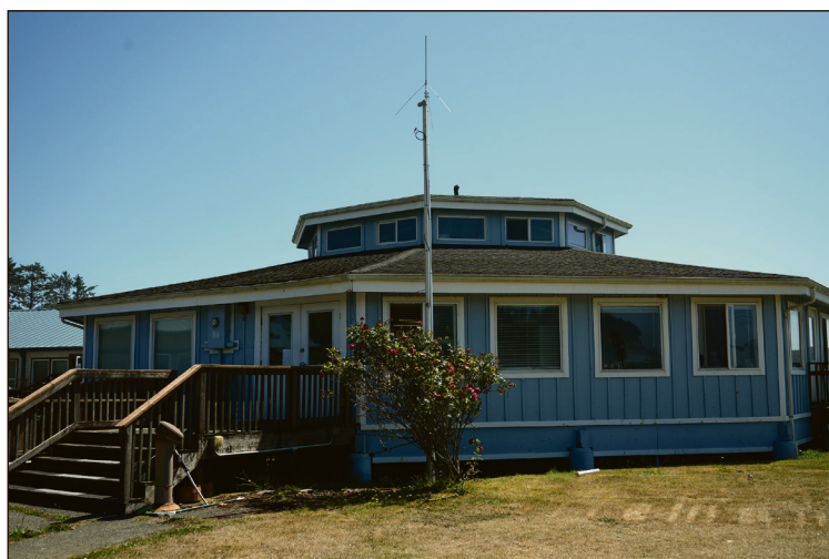
Test installation at the Roundhouse.
